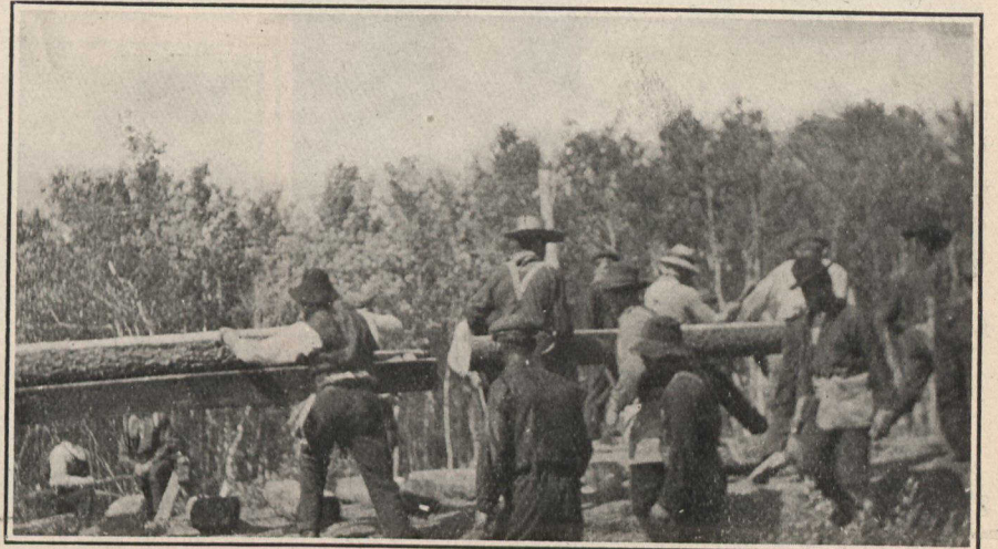
Tie Buckers putting down ties at the rate of 20 a minute
