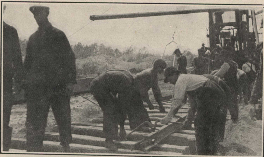
The Pneumatic Lifter lays the rails on the ties
