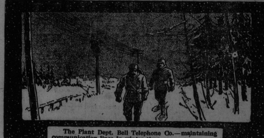
The Plant Dept. Bell Telephone Co.—maintaining communication lines in winter time.
