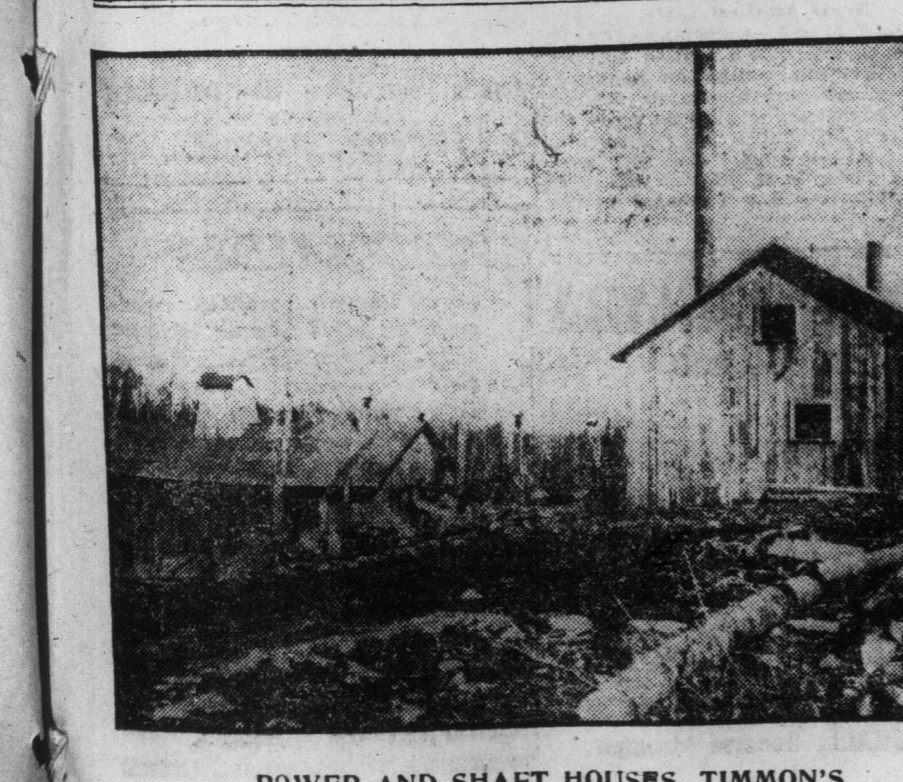
POWER AND SHAFT HOUSES, TIMMONS
