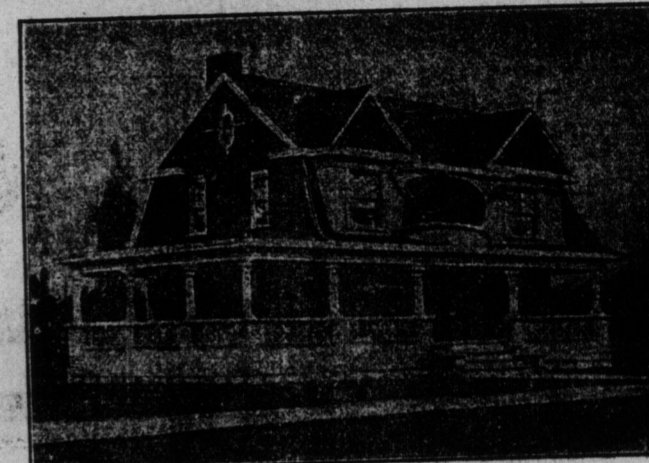
A Park Residence
