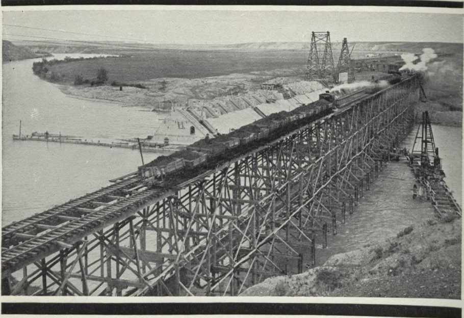
TRESTLE BRIDGE JUST ABOVE THE DAM UNDER CONSTRUCTION
