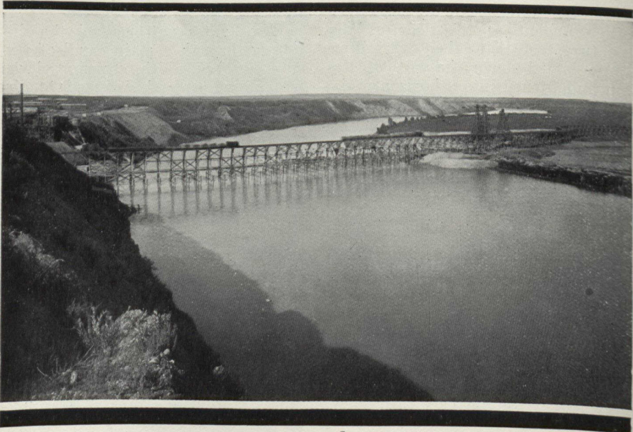
THE BASSANO DAM UNDER CONSTRUCTION
