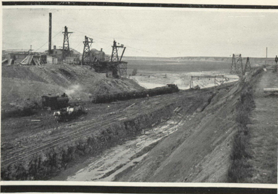
THE ENTRANCE TO THE CANAL FROM THE DAM
