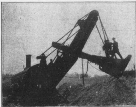
Giant Class E 65-ton, 2-yd. Steam Shovel digging gravel ballast.
