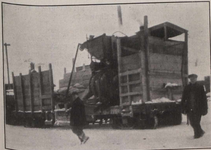
Fig. 1.—Concreting Outfit for Pole Footings.
