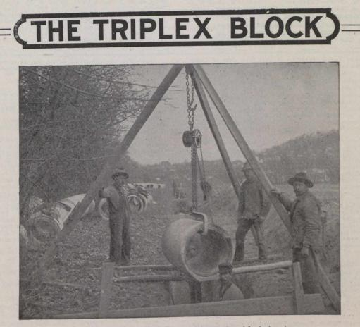
A Triplex Block hung from a temporary rigging and used for laying pipe.
