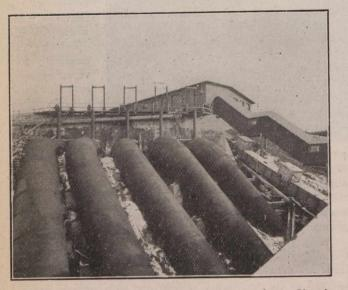
View Showing Penstocks with Cate Mechanisms Showing Above Dam.
