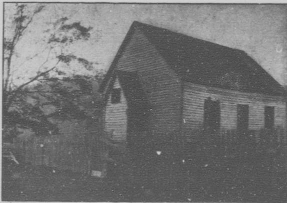
THE FIRST METHODIST CHURCH IN THE CHILLIWACK VALLEY, BUILT 1869
