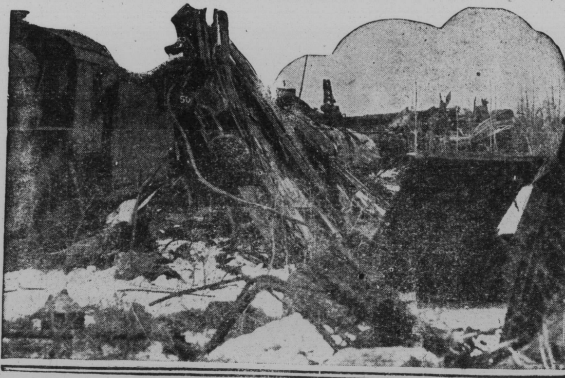
The tangle of wreckage of train No. 4, with wrecking train standing beside it. The remains of the other engine and baggage car of train No. 3 are shown in the background at the right.
