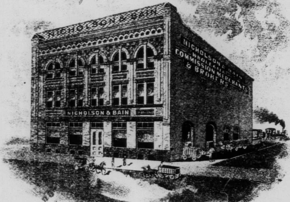
BANNATYNE ST EAST TRANSFER TRACK.
