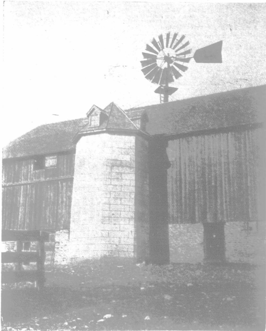
Barn of A. C. Pettit. Silo built with Battle's Thorold Cement. Dimensions 30 feet high and 12 feet in diameter. Driving-house floor 26 x 36 feet.
