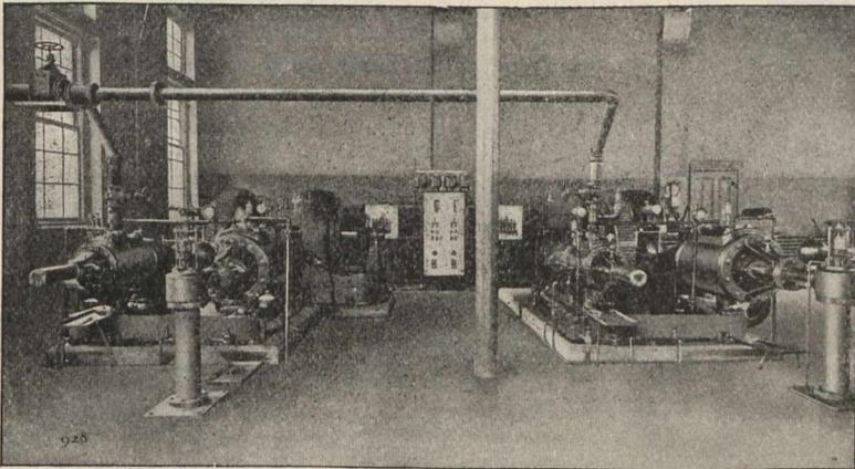
prise the plant. These machines are fitted with modern devices, which contribute to their successful and economical operation. The free air capacity of each unit, running at 130 R.P.M., is 455 cubic feet per minute, and the pressure used is from 70 to 80 pounds.
