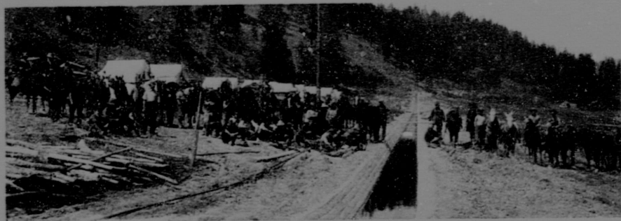
PART OF $300,000 SYSTEM OF CENTRAL OKANAGAN IRRIGATION COMPANY
