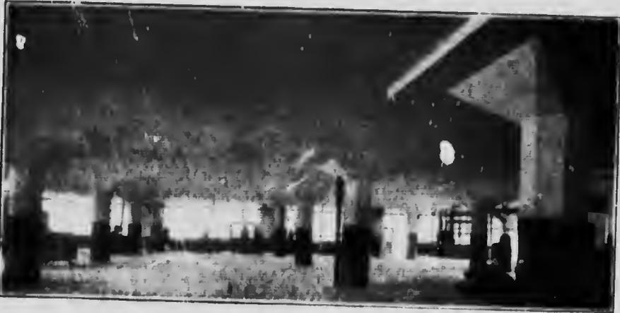
Plant for Graham's Limited, Belleville, comprising warehouse of two stories and basement; cold storage, three stories and basement, and offices of three stories and basement. All built of reinforced concrete. Total cost \$160,000. The entire plant erected in three months.
