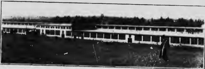
Munition Plant for Pembroke Iron Works at Pembroke, Ont., size 142x160 ft., including heatroom of 110x142 ft., containing 55-foot trusses. Cost \$85,000.00. Plans were made, materials ordered, and building erected in thirty working days.
