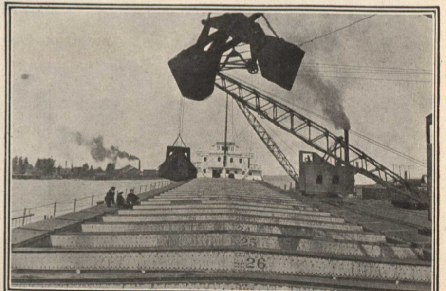
Forward over the hatch-ways of a 550-foot vessel unloading ore at Pt. Edward.
