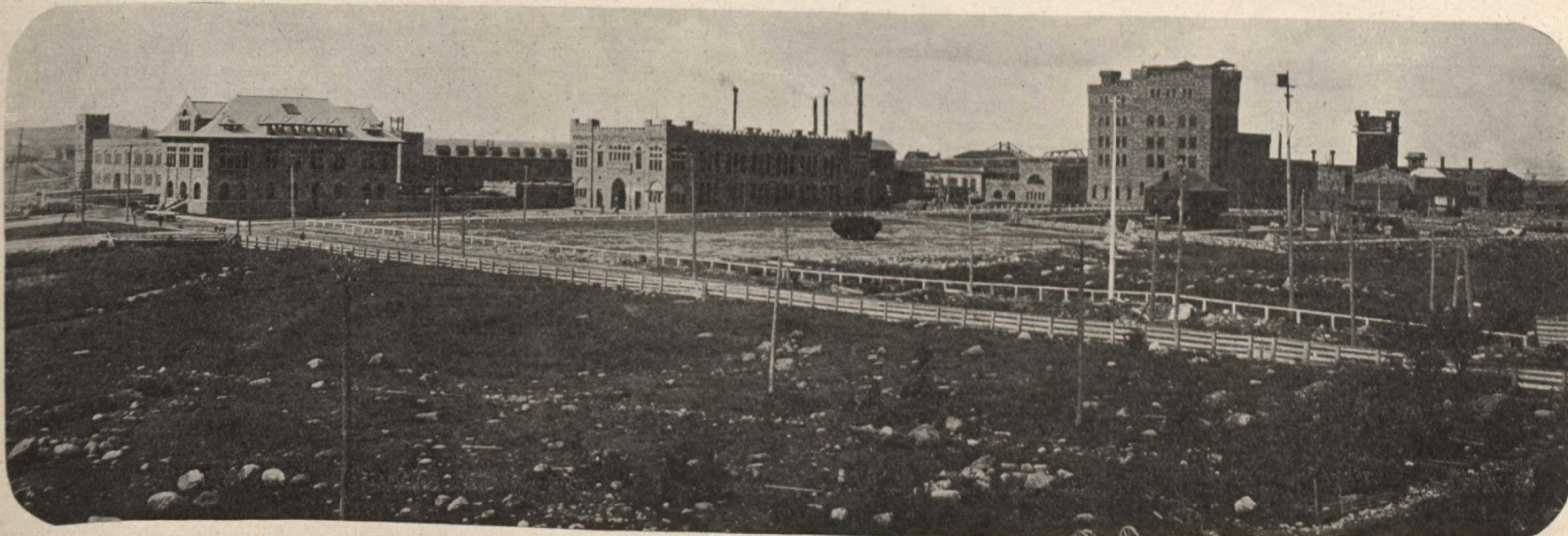
The Lake Superior Corporation at Sault Ste. Marie is doing well. In this picture are shown the General Offices, the Iron Works and the Pulp Mills
