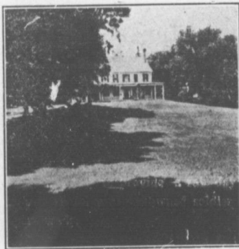
Paint on the shutters, doors and windows, climbers around the verandah posts, a stretch of lawn and a few trees make this old frame farm house a very pretty and comfortable home.
