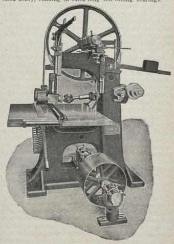
No. 202 Band Rip and Edging Saw. Manufactured by J. A. Fay & Egan Co., Cincinnati, Ohio.
