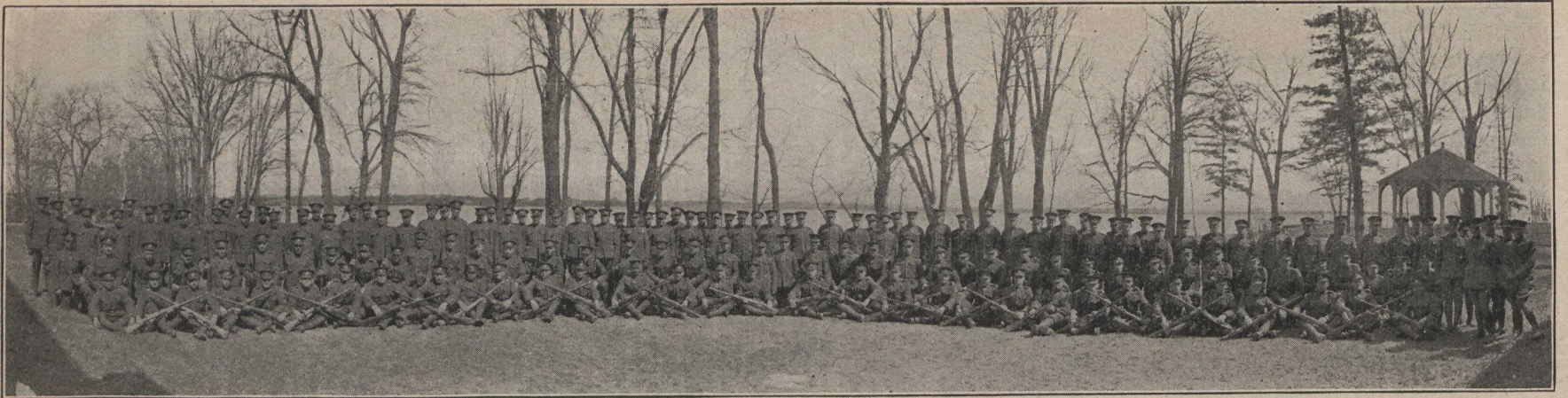
Sections 1—6 (incl.) Base Coy. Engineer Training Depot, St. Johns.
