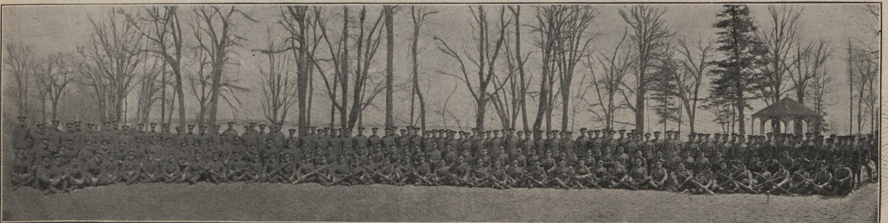
Sections 7—12 (incl.) Base Coy. Engineer Training Depot, St. Johns.
