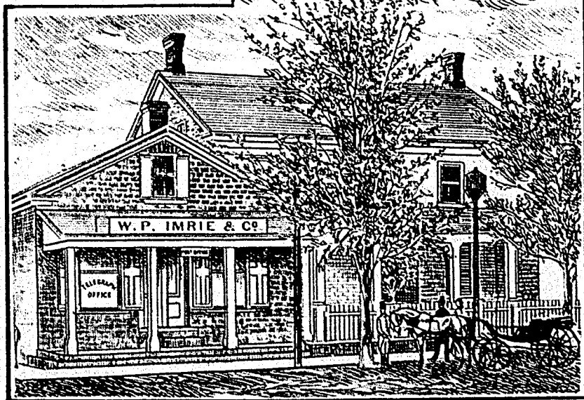
MESSRS. W. P. IMRIE & CO., STORE AND RESIDENCE.
