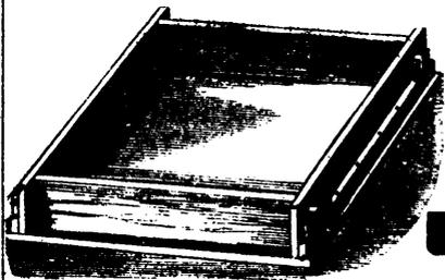
Fig. 1.—BOX FOR MIXING CEMENT.
