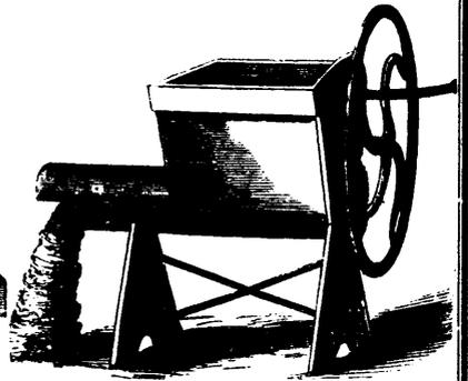
Fig. 5.—MACHINE FOR MIXING CEMENT.
