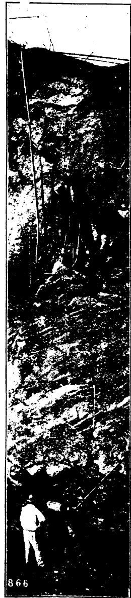
Sergeant "Auxiliary Valve" Drill at work in rock excavation. For all its various uses see our Catalogue No. 81 just issued.
