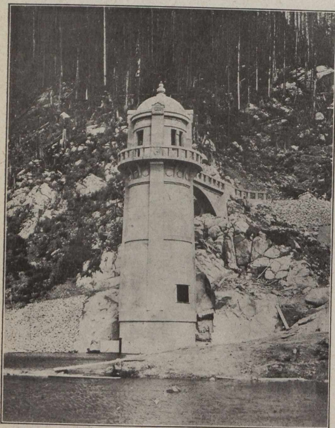
Intake Tower, Coquitlam Lake, New Westminster Waterworks, B.C.
