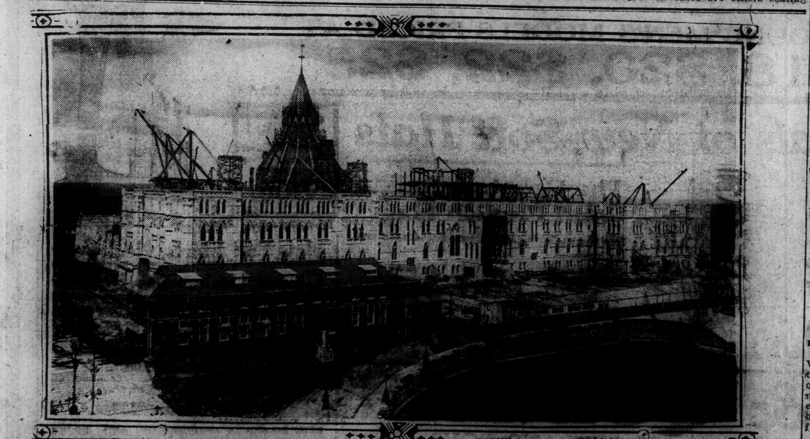
CANADA'S HOUSE OF PARLIAMENT RISING FROM ITS ASHES. A year ago to-day the bits of the Parliament Buildings in Ottawa was a scene of desolation. The ruins of the tower were all that remained of the blackened site. The photograph shows what transformation a year has brought. Only eight months have been spent in construction however, as nothing was done in the winter months.
