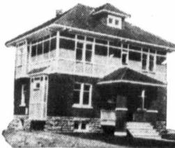
Residence at 295 Clew Avenue, Ottawa. Bishopric Stucco Board used on all interior and exterior walls. Plastered inside; brick veneer first floor and stucco second floor outside.
