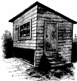
Fig. 12.—Scratching Room Under Poultry House.
