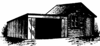
Fig. 2.—Implement House Transformed into a Poultry House.
