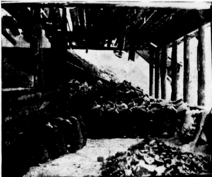
INTERIOR OF ORE SHED, HEWITT MINE, AT NO. 3 TUNNEL.
