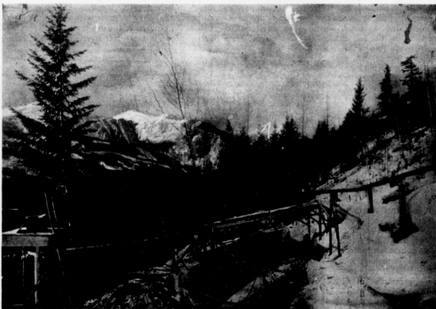
WATER-SUCTION BLAST FOR THE VENTILATION OF TUNNEL. IN OPERATION AT EMILY EDITH MINE, NO. 1 TUNNEL, NEAR SILVERTON.
