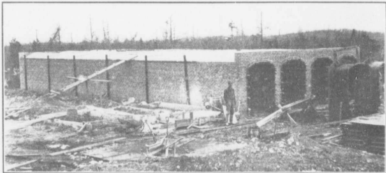
Newington peat works, under construction.
