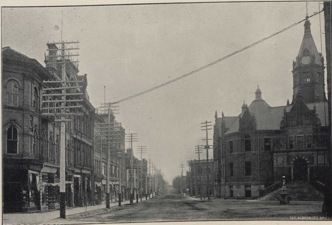
AN EARLY MORNING VIEW ON DOWNIE STREET
