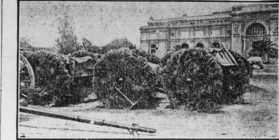
The excessive heat of the summer sun in Egypt and other places of similar latitude has an injurious effect upon artillery, especially upon the tires of wheels, and these, as our photograph shows, are covered with straw to protect them from the sun. The photograph was taken in the square of the famous Kasr-en-Nil Barracks at Cairo. Similar coverings for artillery are, of course, used in the field as a disguise to conceal the position of guns from hostile aircraft. Recent war news from Egypt has concerned chiefly the accommodation of wounded and prisoners from the Dardanelles, and has recorded no further attacks on the Suez Canal. It was reported recently from Cairo that most of the Turkish forces in Sinai and Syria had been withdrawn to assist in defending the Dardanelles.
