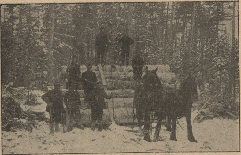
A Skidway in course of erection.
