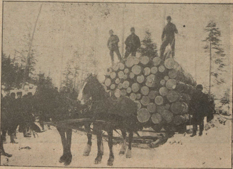
A completed load ready to be taken to the "dump."
