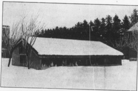
Twenty feet square, open front Poultry House. Good ventilation, but no draught.
