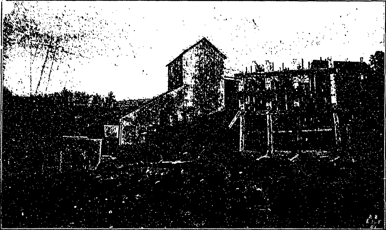
Oldham Gold Co.—Exterior of Mill Building with Battery of an old Mill in front, at Oldham, Nova Scotia.
