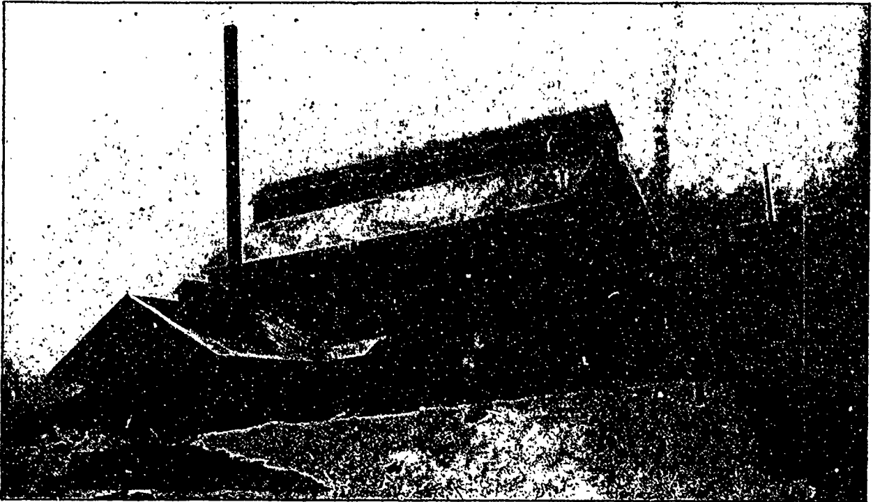
Bell's Asbestos Co. Ltd.—Exterior of Mill Building, Thetford Mines, Que.
