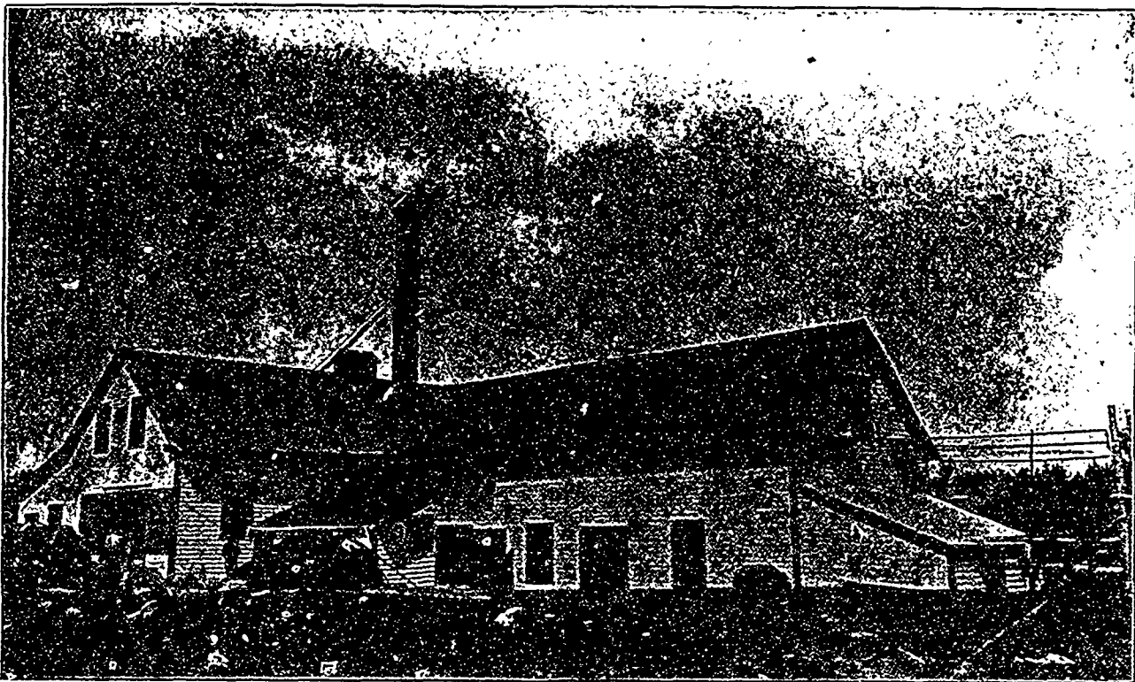
Golden Group Mining Co.—Exterior of Mill Building at Montague, Waverley District, Nova Scotia.
