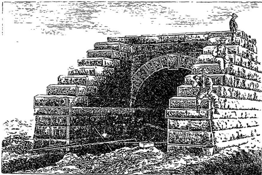
FIG. 3.—CULVERT UNDERNEATH EMBANKMENT.—INTERCOLONIAL RAILWAY.
