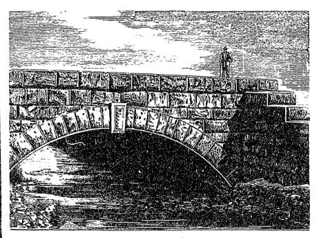
Fig. 4.—Segmental Arch Culvert.—Intercolonial Railway.
