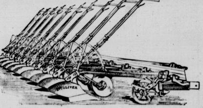
Oliver feature is a hitch which enables the horses to be worked four abreast and all walking on unplowed ground, eliminating side beam strains which quickly put a plow out of adjustment. The foot lift is so placed that the operator can quickly place his whole weight on the lever in lowering bottoms. All levers are easy to operate.
