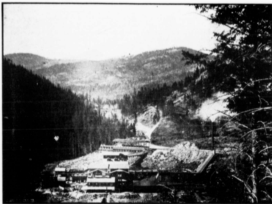
General View B. C. Copper Company's Smelter at Greenwood.
