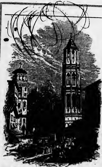
LEANING-TOWER OF SAN-FELIPE CHURCH, SARAGOSSA.
