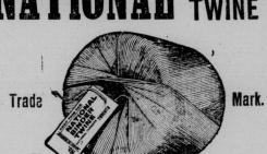
Full strength: over 75 lbs breaking strain. Full length: 600 feet to the pound. Eull weight: 80 lbs to each bale. No clogging in the binder—compactly wound.
