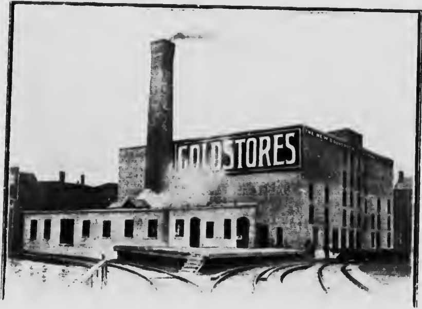
FROM THE UNION STATION, SHOWING SIDINGS, PLATFORM AND POWER HOUSE.
