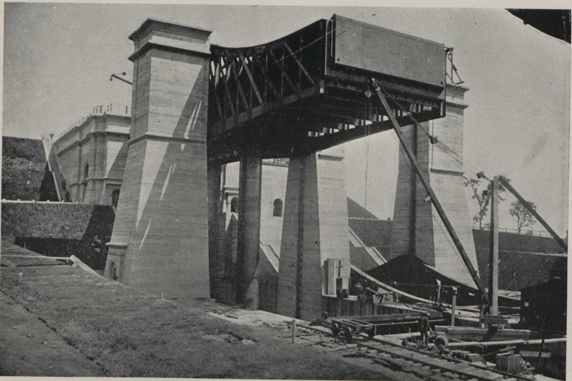
LIFT LOCK NEAR PETERBORO' ONE OF THE PONTOONS AND THE PISTON ON WHICH IT IS SUPPORTED
