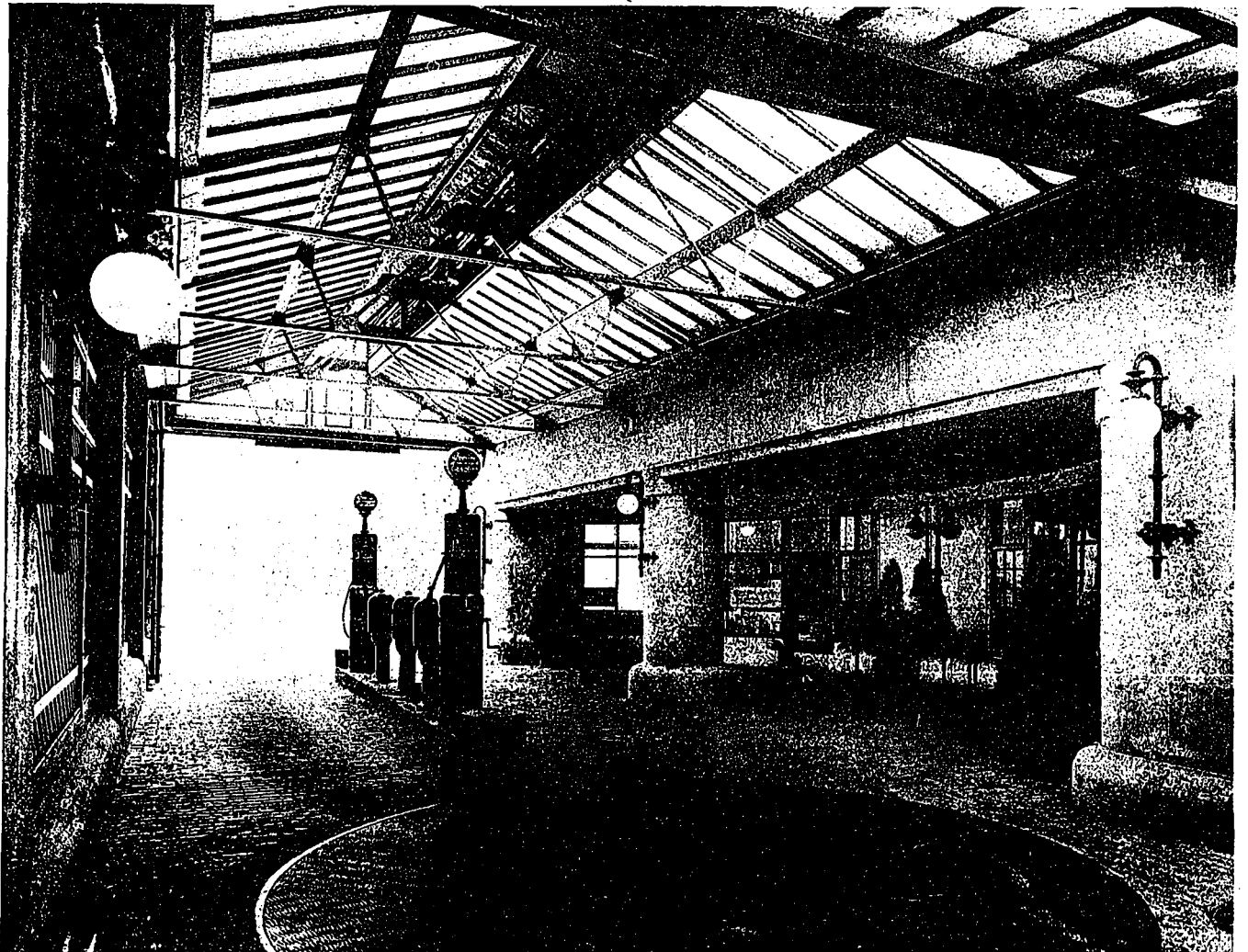
VIEW OF SERVICE STATION, SHOWING TURN TABLE, OIL AND GASOLINE PUMP, IMPERIAL OIL BUILDING, TORONTO, ONT.
