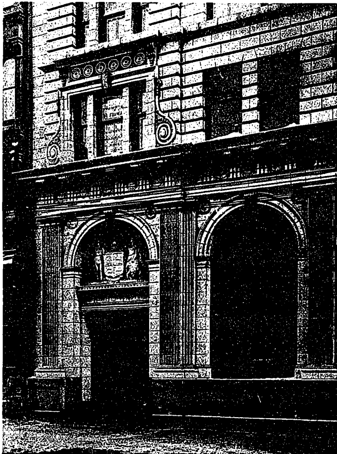
DETAIL VIEW OF MAIN ENTRANCE.
