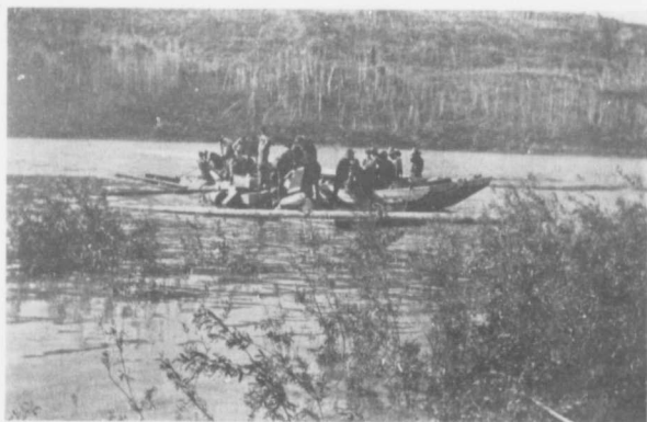
Towing the Wrecked Barge Ashore
