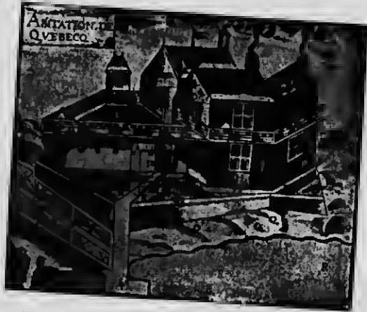
A. Store-house. — B. Dove-cot. — CD. Main Building. — E. Dial. — F. Forge. — G. Gallery. — H. Champlain's Apartments. — I. House-door and Drawbridge. — L. Walk ten feet wide. — M. Ditch. — N. Platform for canon. — O. Champlain's Garden. — P. Kitchen. — Q. Open space reaching to the River. — R. River St. Lawrence.
