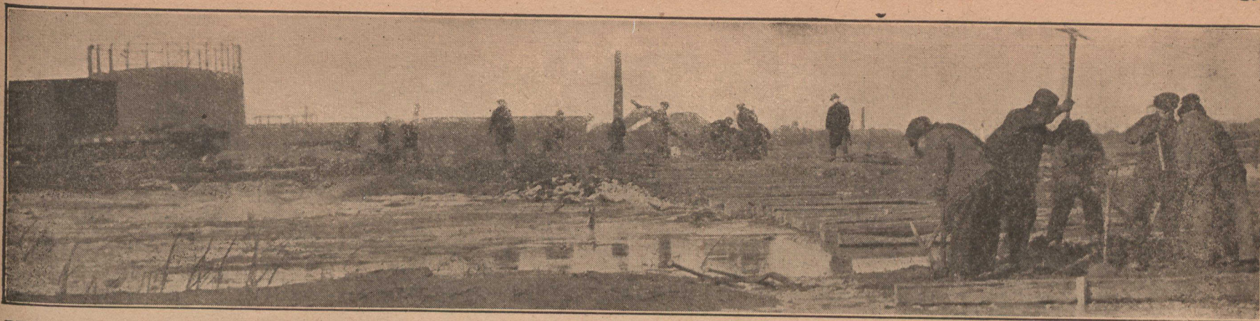
WHERE these men are working—it's the east end of Toronto—was once a useless marsh. The Toronto Harbour Commission took hold of it and filled it with sand pumped up from other parts of the waterfront, where deeper water was required. Now a three million dollar munition plant is being erected where once only cat-fish roamed and bull-frogs sang. The men in this picture are laying a railway siding to carry in building materials.
