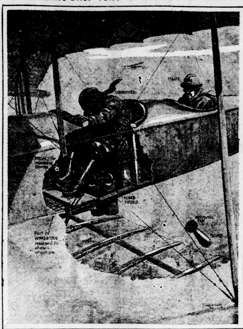
This picture shows the "Roland" bomb-dropping apparatus as worked from a German airplane. The apparatus, which weighs 15 pounds, consists of bomb tubes, tube covers and pedal board, so arranged that the observer may operate with his foot.—Drawn by D. Macpherson in the London Sphere.
