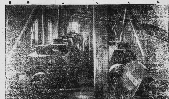
This picture shows one line of Grinding Mills in the "A" side of "Queen City" Mills. Each machine in the picture is fitted with two pairs of solid steel corrugated rolls measuring thirty inches long by ten in diameter. These machines run night and day almost the whole year round making
