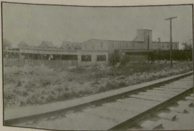
FACTORY OF ROMAN STONE COMPANY, LIMITED. TORONTO, ONT.
