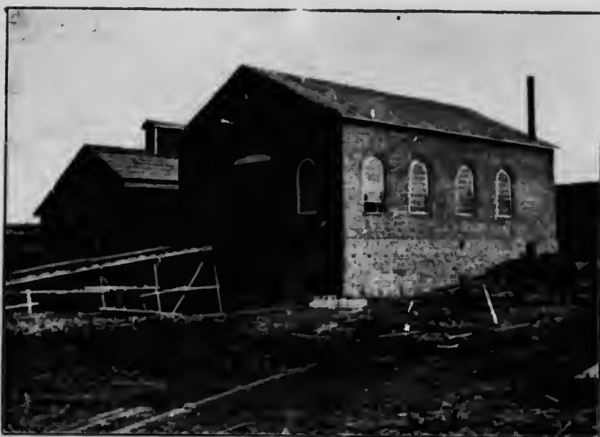
BOILER ROOM AND ENGINE HOUSE OF SUBMARINE HOISTING PLANT.
